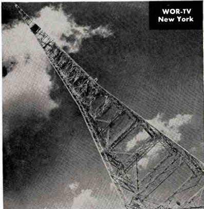
WIND LOADING 60 POUNDS! Rising 1050 feet above the Hudson River, the WOR-TV tower at North Bergen, N. J. is the highest structure in the state. General Electric FM and TV antennas, mounted together on a special mast, can resist a wind velocity of 165 mph. WOR-TV is also equipped with General Electric FM and TV transmitters and a custom built control console.
